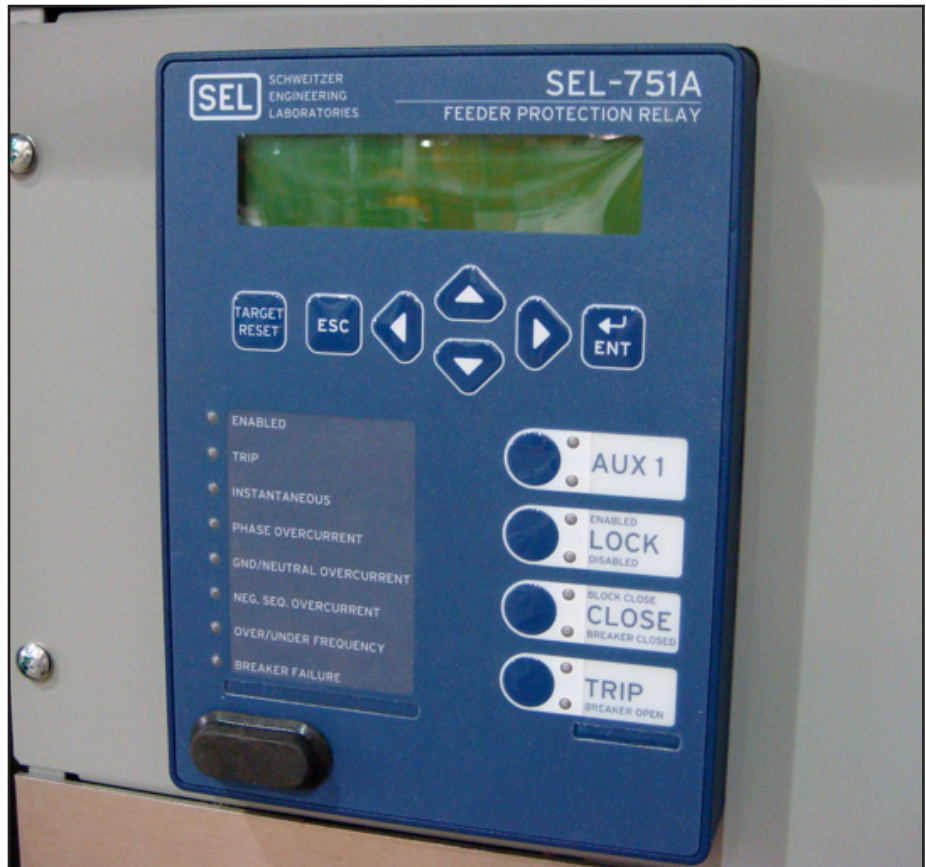
▲ Schweitzer's SEL-751A control is one of many control options.
