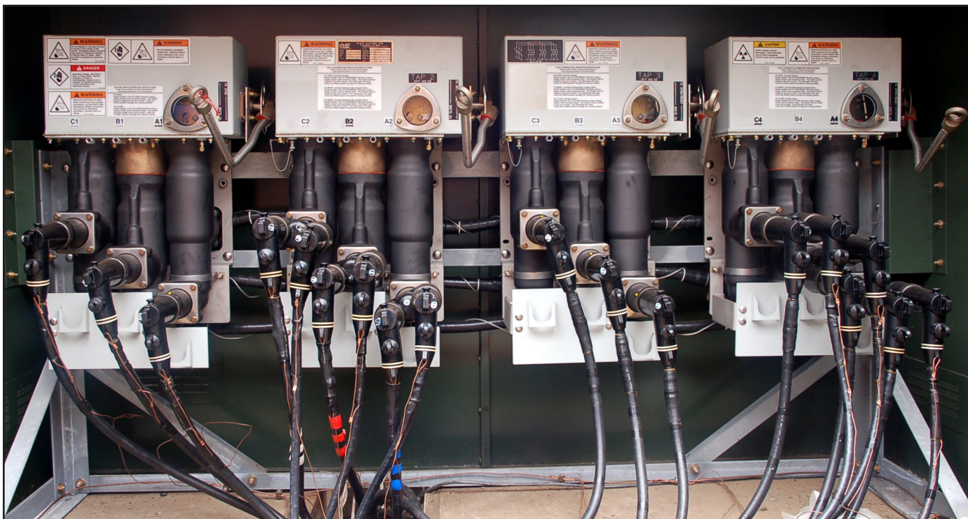
▲ Four-way front access, padmount Trident-S.
