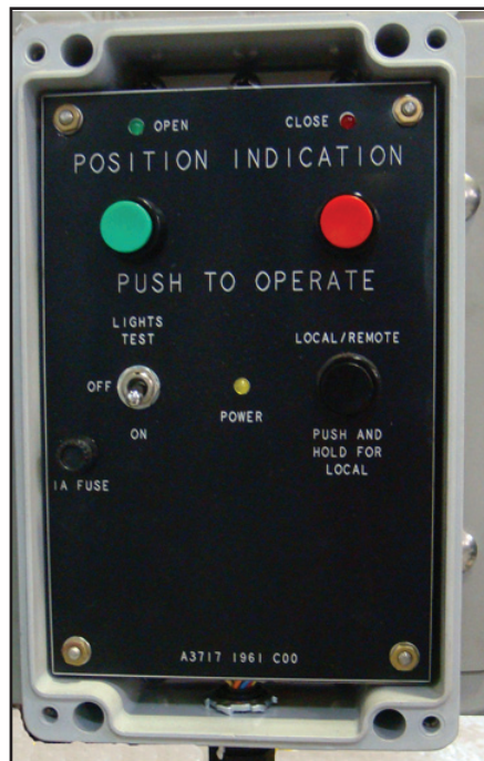
▲ Stationary controls permit either local or remote SCADA operation.
