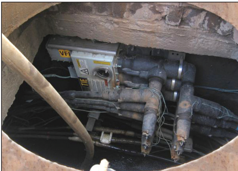
▲ Three phase Trident-S fault interrupters in a submersible vault application.
