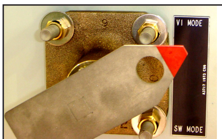
▲ Load Break / Fault Interrupter Selector Switch
