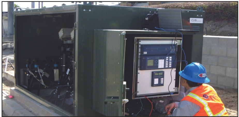
▲ Padmount switch with SEL controls.
