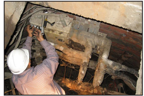
▲ Horizontal mounted fault interrupter in a submersible vault.
