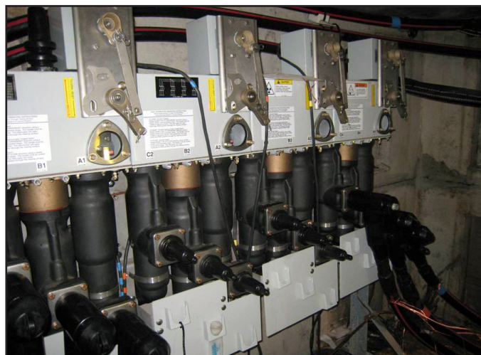
▲ Automated multi-way, Trident-S in a submersible vault installation.
