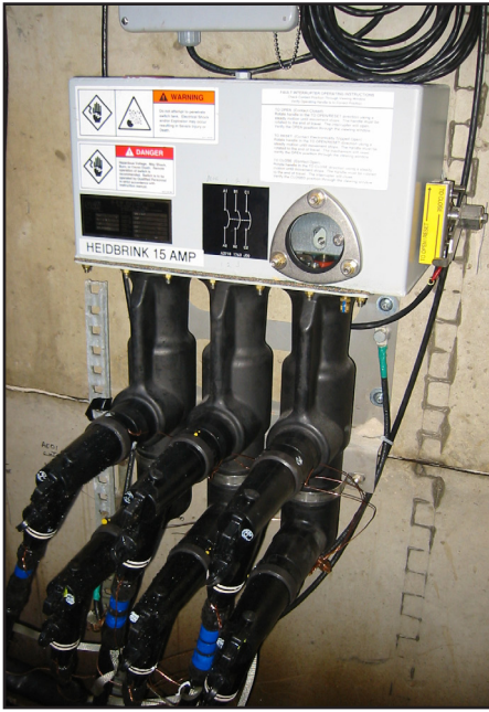
▲ Fault interrupter with wall mounted control box and side mounted operating handle.
