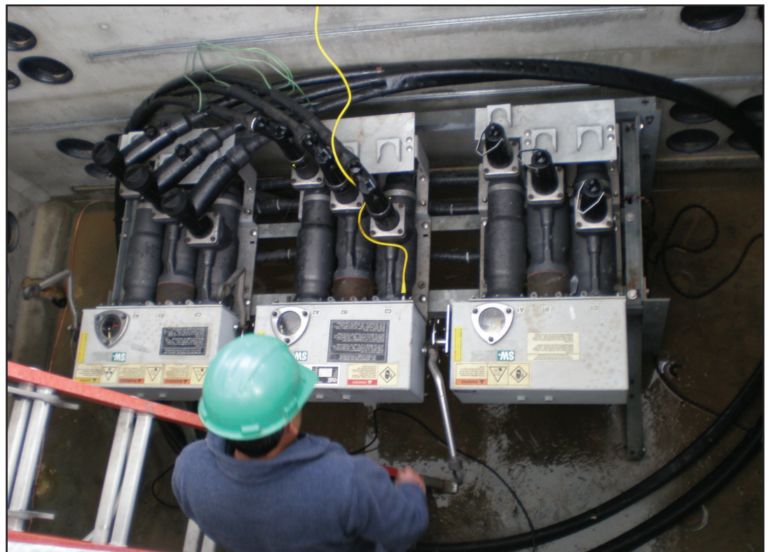
▲ Three-way, submersible vault, automatic transfer switch including submersible G&W ATC451 control.
