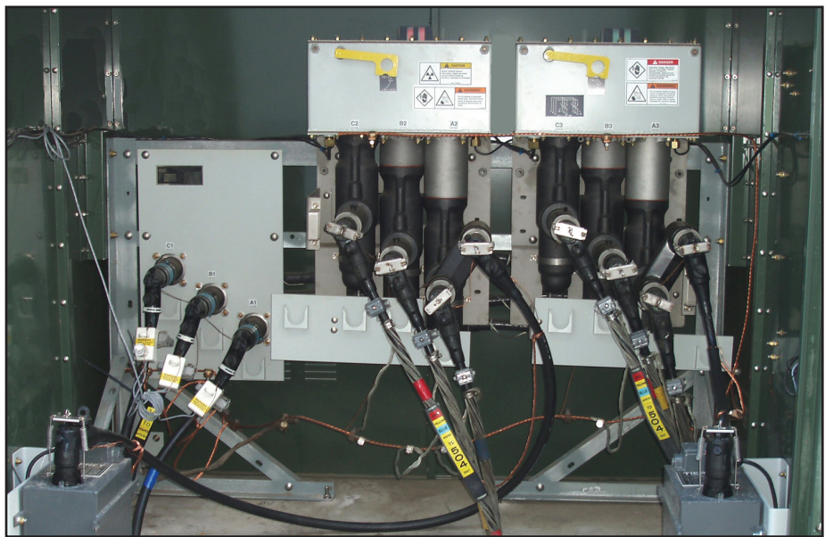
▲ Automated padmount switch utilizing magnetic actuators and integral voltage sensing electronics for a high speed automatic transfer application.
